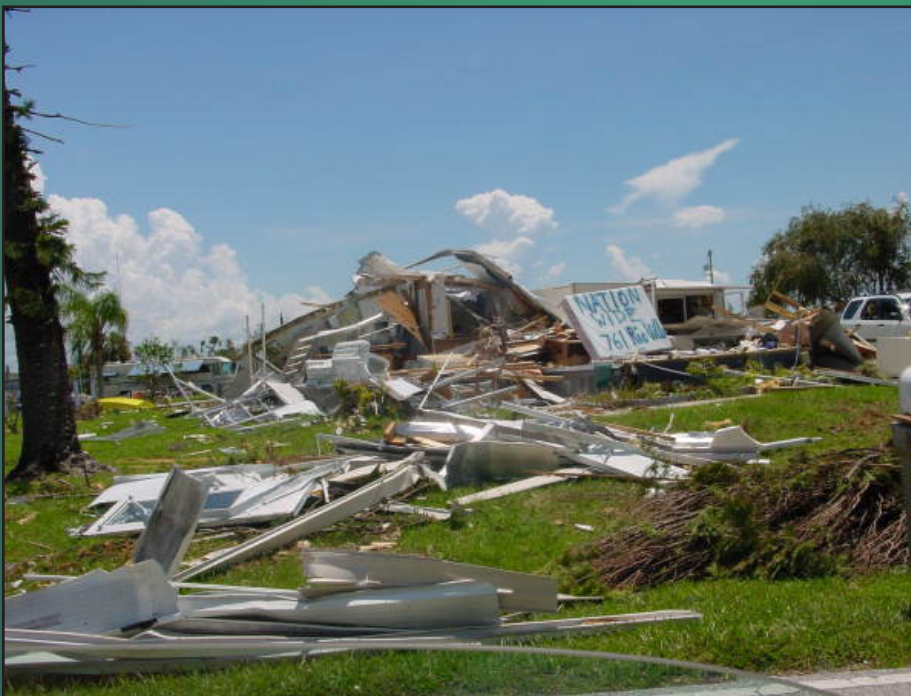
Figure 9. Hurricane Charley damage, David Bujak, Florida Memory.
